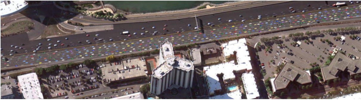
Figure 1: The divided highway is populated with vehicle traffic using our flow reconstruction method. Individual virtual cars are animated and correspond to real-world traffic conditions measured by road sensors. The vehicle motions are simulated on a GIS-derived domain and overlaid on a public domain aerial image from the U.S. Geological Survey.
